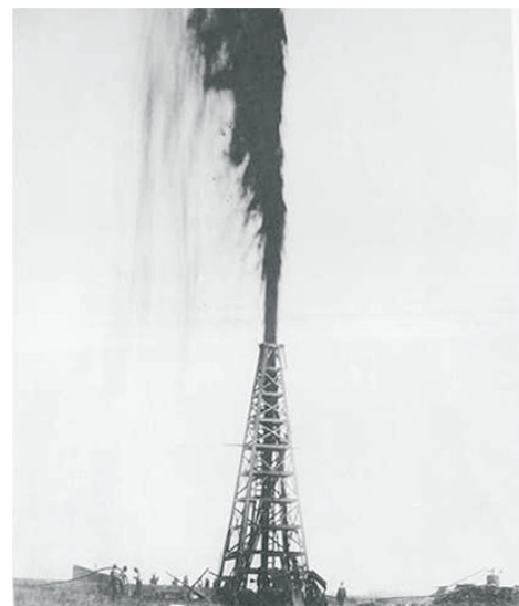
Spindletop gusher 1901. Original photo by John Frost.
